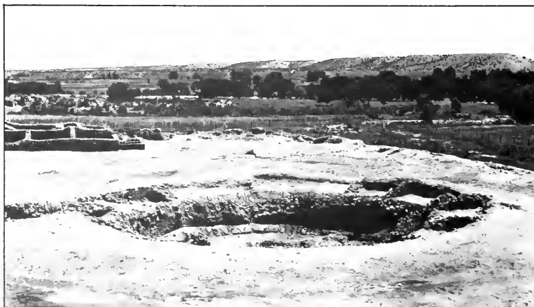
Figure 7.9. Deteriorated condition of Great Kiva prior to reconstruction in 1934.
